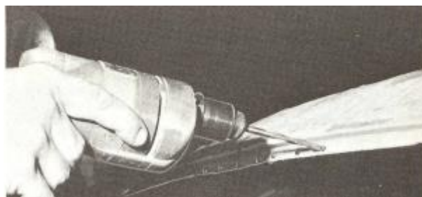
Figure 2- 40 Drilling out spot welds at front edge of roof
