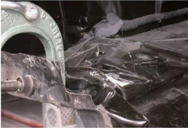
A This panel has been kinked and badly damaged. A frame rack has been attached to the panel for pulling, even though the panel will be replaced.
