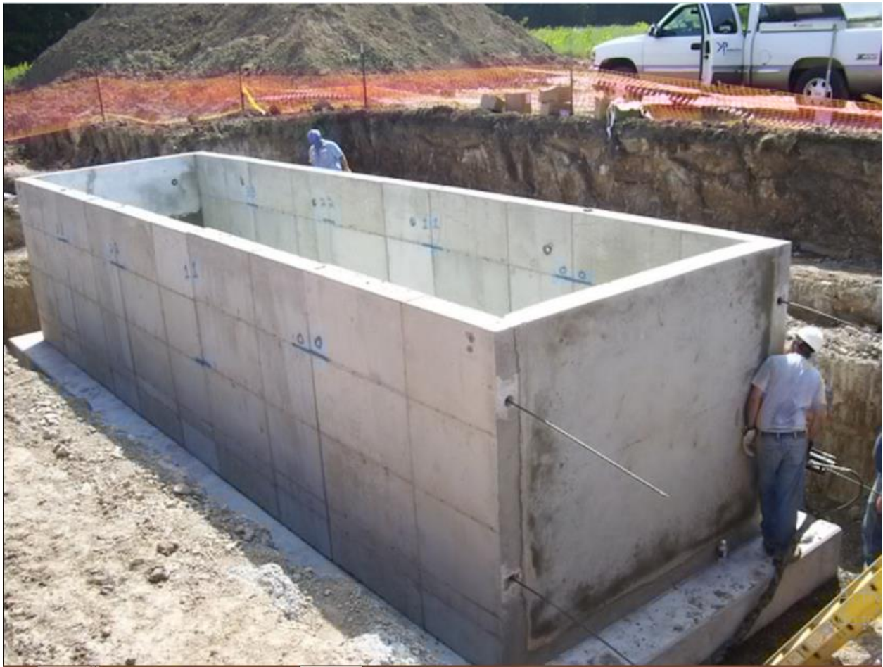
Fig 2.2 concrete septic tank
