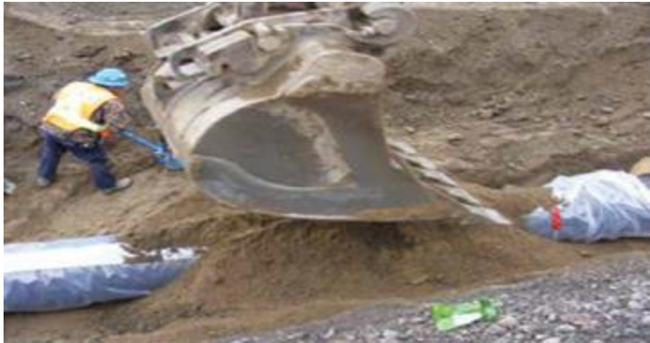
Fig 5.3 Backfilling the excavated soil
